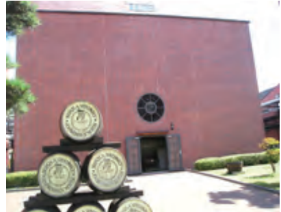
Repair and protection of exterior wall tiles
