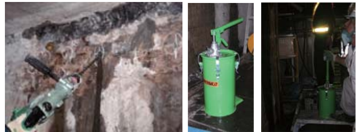
There are more than 20L. of water leakage per minute from this area
