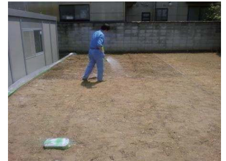
The application amount is scattered on the basis of 2 kg per square meter.
