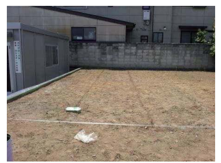
Secure construction area with rope
