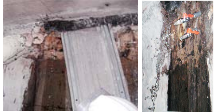
There are more than 20L. of water leakage per minute from this area
