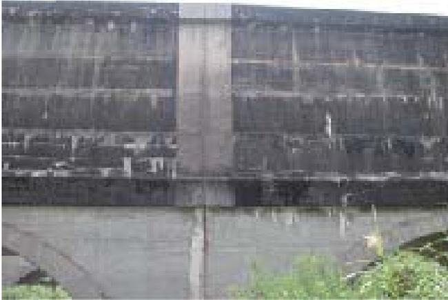
**As deterioration by the alkali aggregate reaction progresses, the concrete structure,**
