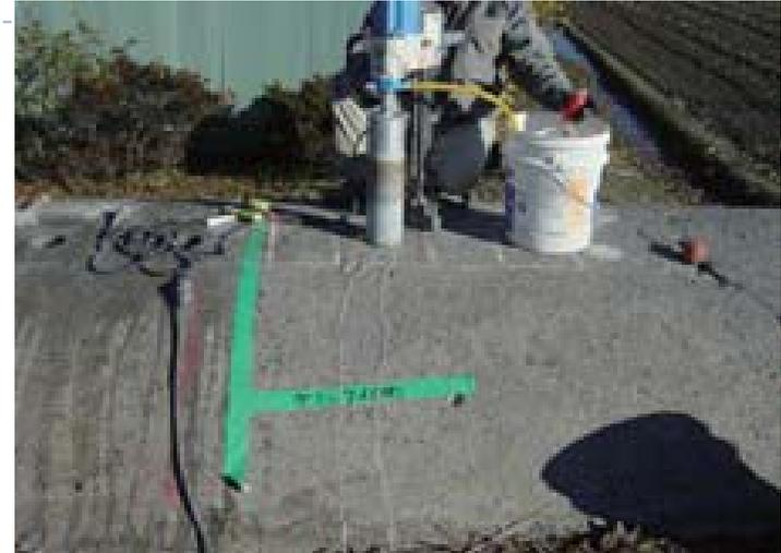
Cut the concrete with diamond core drill of 10 cm long while sending water with a pump.
