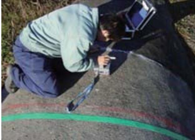
Before construction, check the position of the interior reinforcement and open the core while sending fixed water to the core drill.
