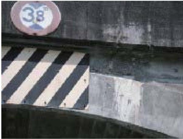
Collect cores and investigate whether alkali-reactive aggregate is used or observation with polarizing microscope.
